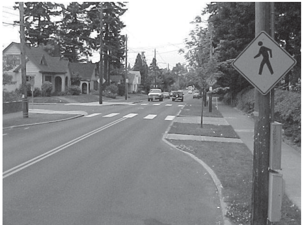
Curb extensions (above) reduce crossing distances for pedestrians and can calm traffic.
